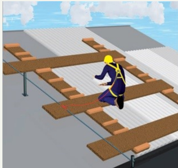
Preparation of the board with a lifeline fall arrest system.
