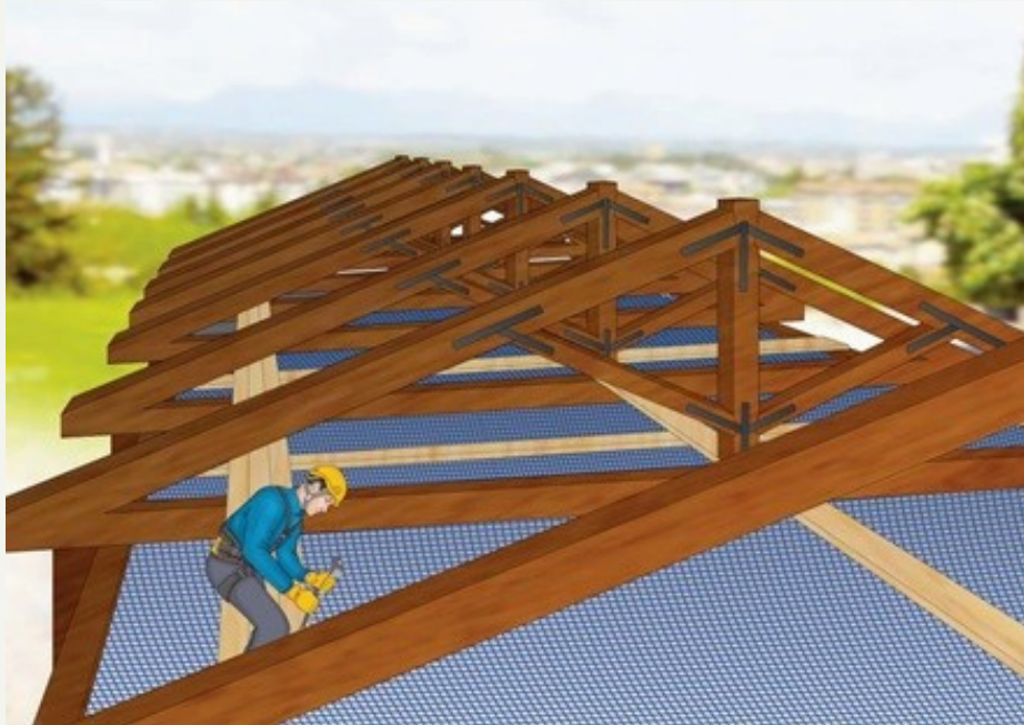
Operator connected to fall arrest system (lifecycle, harness, etc.), preparation of walkways with boards, and utilization of safety nets (System S).
