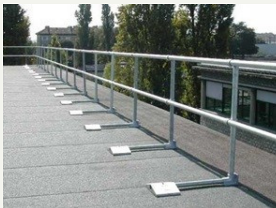
Roof safeguarded by parapets
